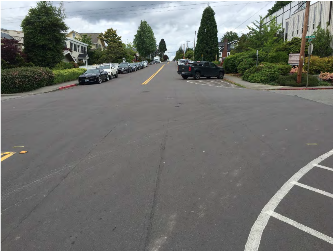
Figure 5. Example of slurry seal applied in nearby Kirkland, WA.
