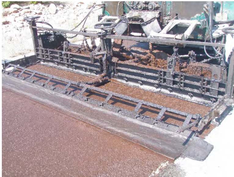
Figure 6. Example of micro surfacing application.
